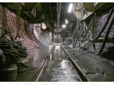
Tunnel section with location of the shot holes on the left hand side of the tunnel and the localised inflow of water.
