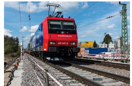
Tracks in the section of Tunnel Rastatt
