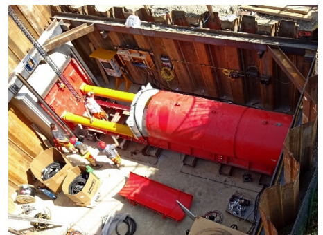
Start shaft of the micro tunneling
