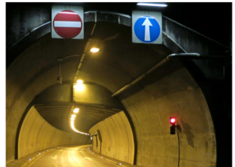
Mositunnel with intermediate ceiling
