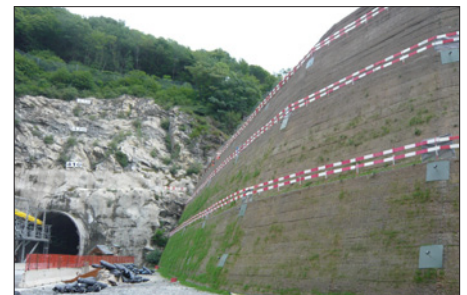
Wall of reinforced soil
