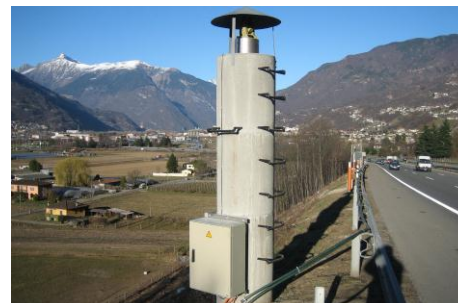
Pillar with total station
