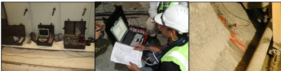
TSP system on TBM site Site geologist at TSP work TSP receiver set 2m deep
