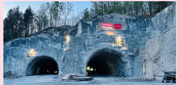
Entrance to Bjønnås. Twin tube tunnel under construction
