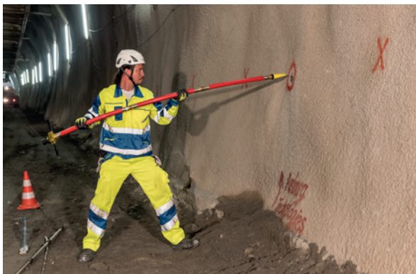
Like a rock bolt: Simple installation of seismic receiver unit
