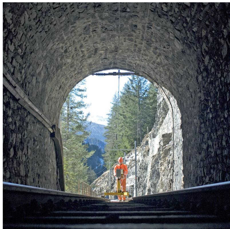
Thanks to the use of cutting-edge laser scanning technology, it was possible to survey almost all tunnels on the Rhaetian Railway in a short time in 2006 and 2007 (31.2km excluding the Vereina line). The digitalised data opens up new possibilities for selective deployment of resources.
